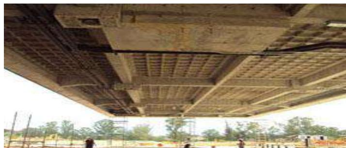
Figura 6: Lajes nervurada
